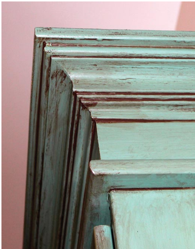
Inexpensive MDF was used to add trim and mouldings for added style
