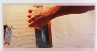
**Step 5** Using the 3/16" v-notch trowel on about a 45-degree angle, spread the adhesive to a uniform thickness and consistency.
