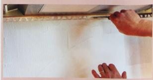
**Step 7** You may use a tile trim at the end where tile transitions to wall. Wait 24 to 48 hours before grouting. For wall tile applications a non-sanded grout with an integrated sealer works best.
