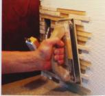
**Step 6** Lightly press the tile into place. Using a grout float with firm pressure will help you achieve a uniform pressure on the mosaic tile. Repeat the process throughout.
