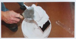
**Step 4** Using the 4" plastering trowel load the v-notch with adhesive. Use the 4" knife to spread adhesive to the wall as evenly as possible. Do not try to work areas larger than you can deal with in 10-15 minutes.
