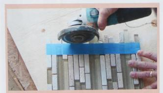
**Step 2** Using a dry saw with a diamond blade, cut one side of the first tile off square to begin your run. Wet saws do not work well with mosaic tile as water affects the mesh backing, as well as the tile glue.
