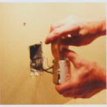
**Step 1** Start by turning off the power to counter plugs and checking to make sure there is no power by using an electrical tick. Unscrew and pull the receptacle slightly out of the box with the power off. Wrap the side screws with electrical tape to ensure trowels and other tools do not come in contact with the wires throughout the process.
